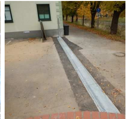
|| Installed condition: Only a drainage channel is visible
