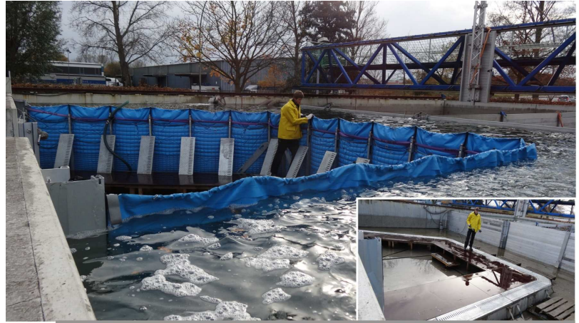
Intelligent Flood Control
