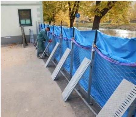
Erected flood wall:
