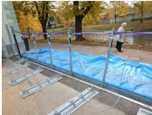
|| - Flood wall in process of erection -
